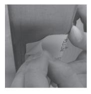
**3.** Carefully cut the frame inside the un-shaded area marked on the template. Install strike per installation instructions 08281280.
