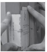
**2.** Peel adhesive backing and paste the folded template square to the frame.
